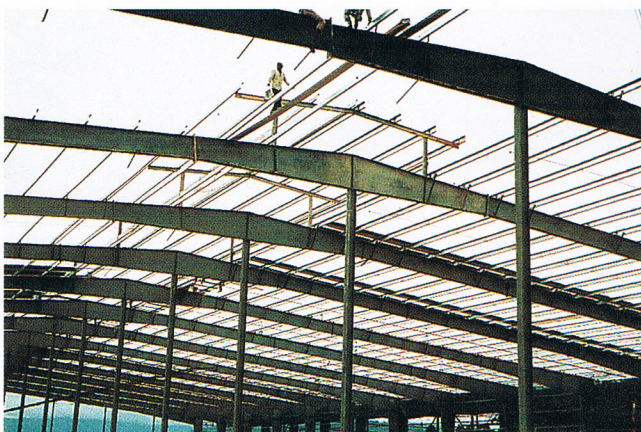
• MEC Factory (Phase I).
