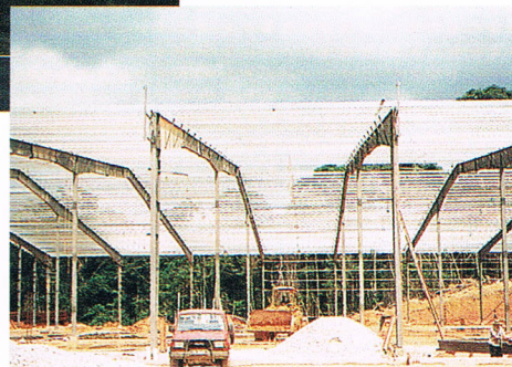
• MEC Factory (Phase II).
